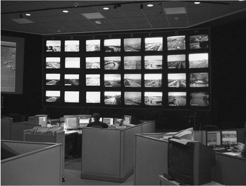
Figure 1. ITS Video Wall for State Department of Transportation
